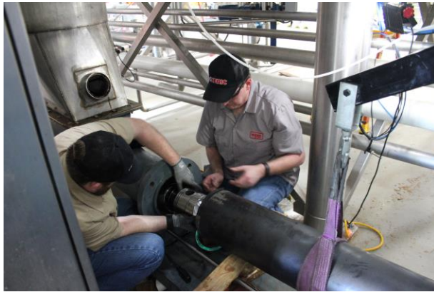
On Site XERIC Upgrade. . .Retrofitted into the existing rubber lined pump.
